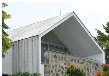
The building. The whole facade and roof treated on the strength of that patch.
