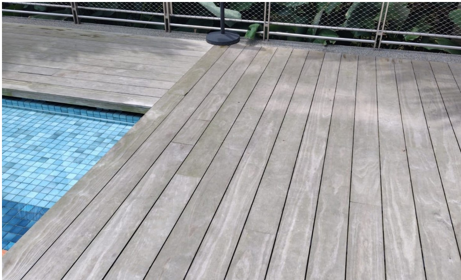
Silicate treated pool deck in service. Grime, salt and light growth accumulate on the surface without affecting the treatment underneath. This is a cleaning job, not a recoating one.
